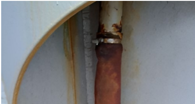
FIGURE 22 Non return valve temporary patch work
