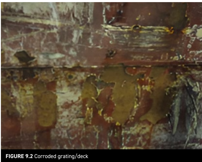
FIGURE 9 Corroded grating/deck
