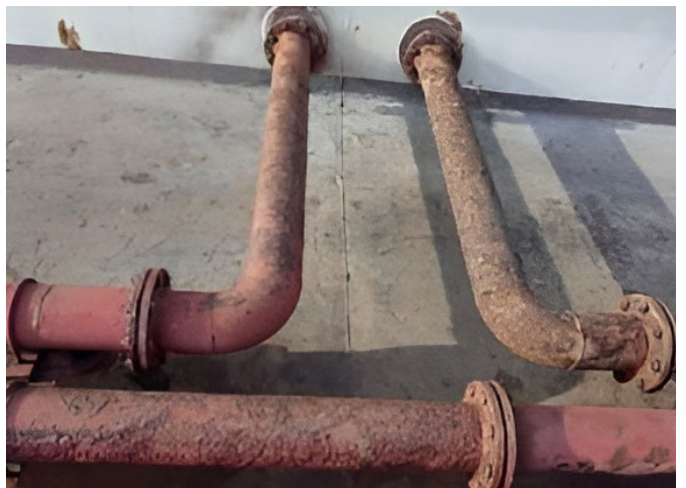
FIGURE 8.2 Corroded pipes
