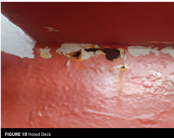
FIGURE 9.2 Corroded grating/deck
