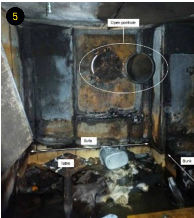
FIGURE 5 AB2'S FIRE-DAMAGED CABIN
