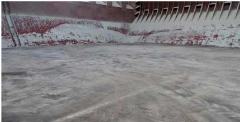
✗ Poorly prepared cargo hold on a bulk carrier. Residue from some bulk cargoes can react with, and damage, steel cargo
