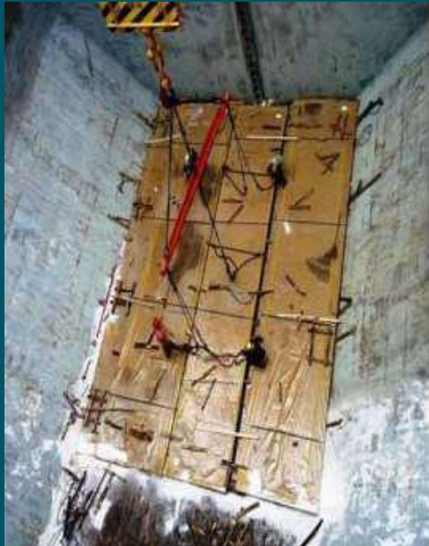
This spreader bar with 3 equidistant lifting slings will reduce plate bending
