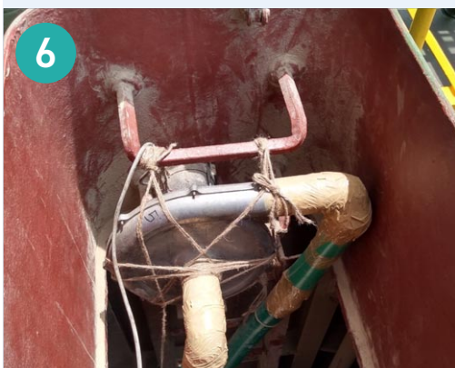
Figures 6: Examples of recirculation fans installed in manholes from different countries - USA and India
