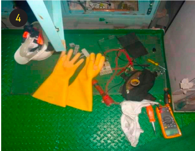
FIGURE 4 TOOLS AND SAFETY HELMET ON DECK WHERE THE ELECTRICIAN WAS FOUND.
