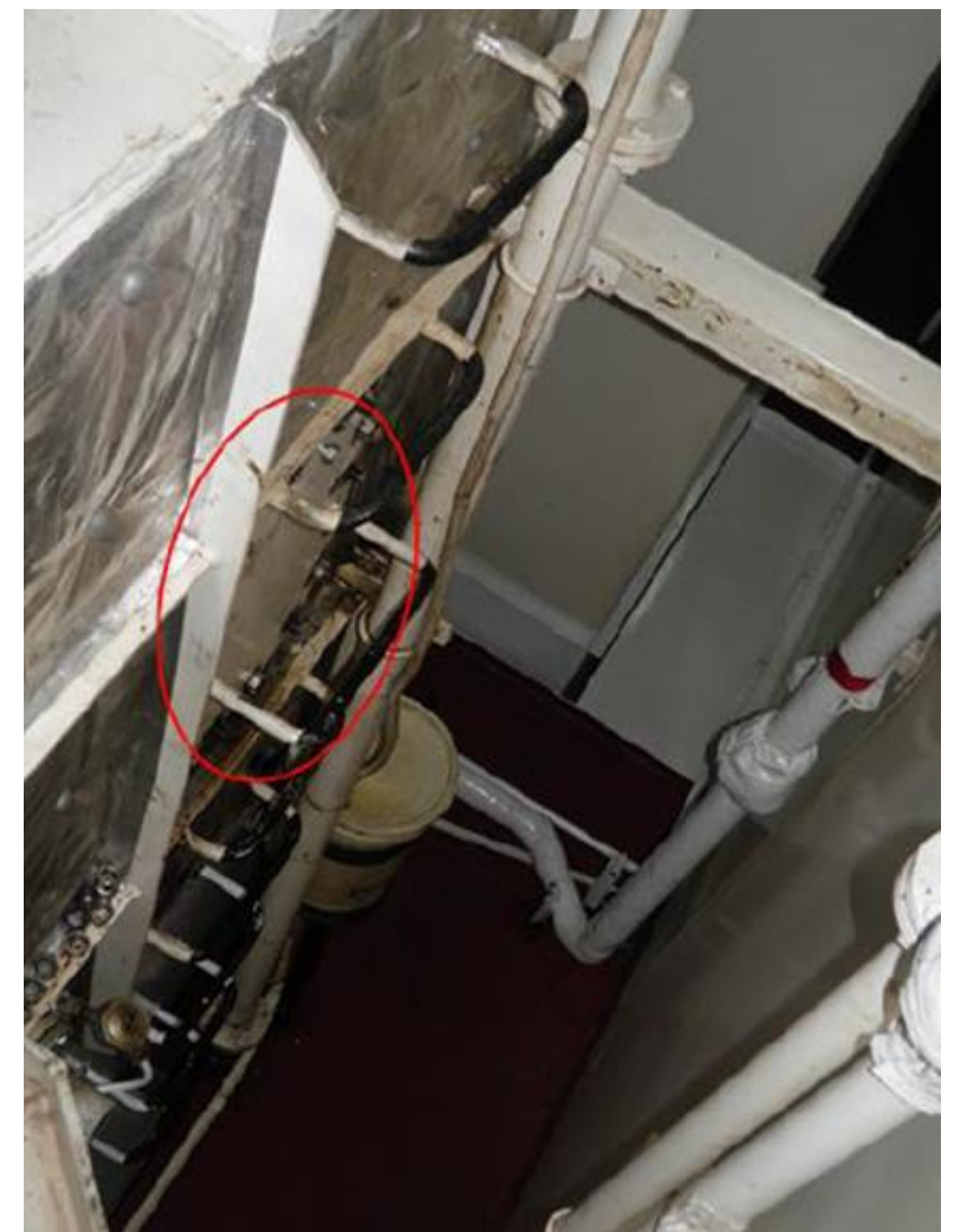
The manhole located two meters from the floor
