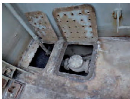
Starboard bilge well
