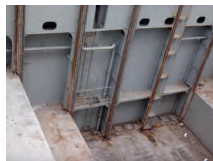
Aft bulkhead of no 4 hold
