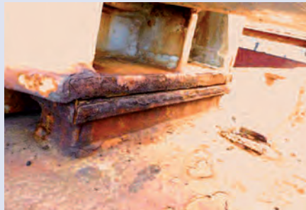
Corroded and wasted hatch cover landing pads.
