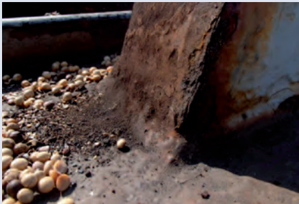
Hatch coaming not swept, cargo debris and rust still evident. Centre line joint closing wedge showing severe wear.
