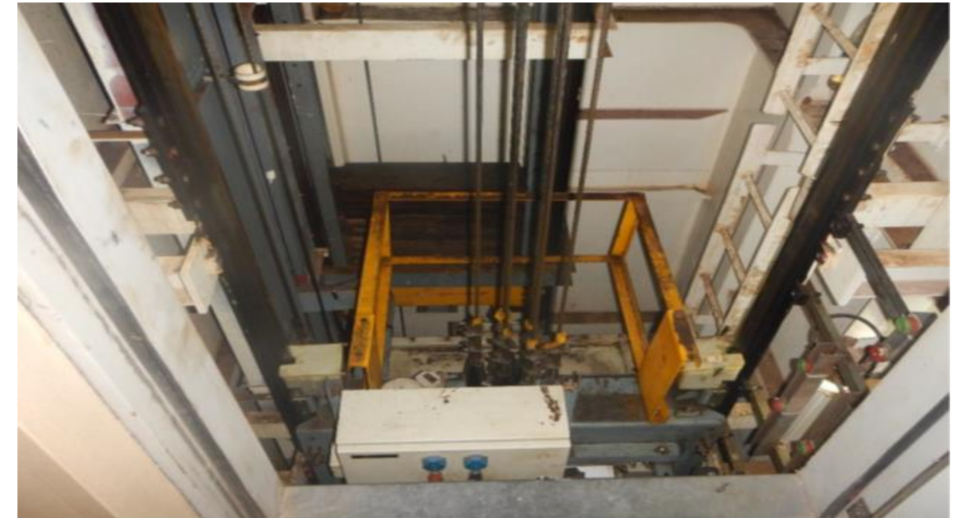
Top of elevator car showing maintenance box and safety cage Source: Investigation report 06/2018 by Transport Malta – Marine Safety Investigation Unit
