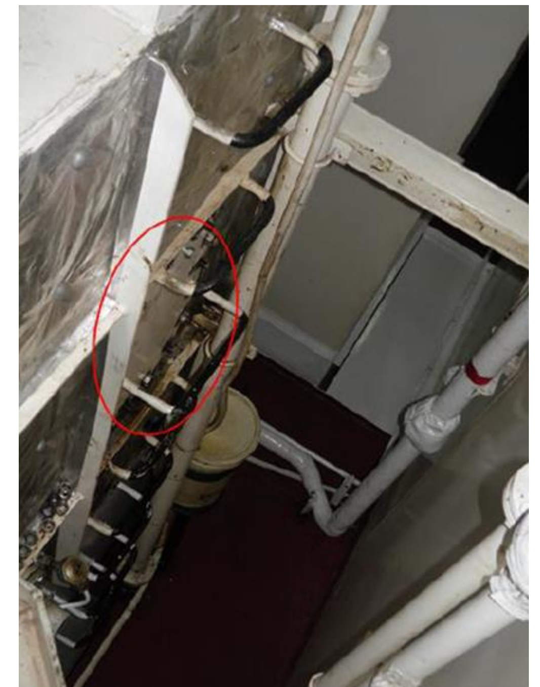
The manhole located two metres from the floor
